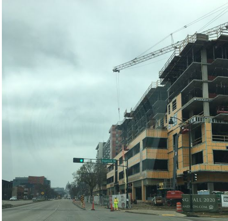
Construction continues in Madison, as it is deemed “essential.”
